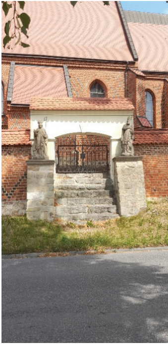
Photograph 2. Contemporary view of the former entrance.
